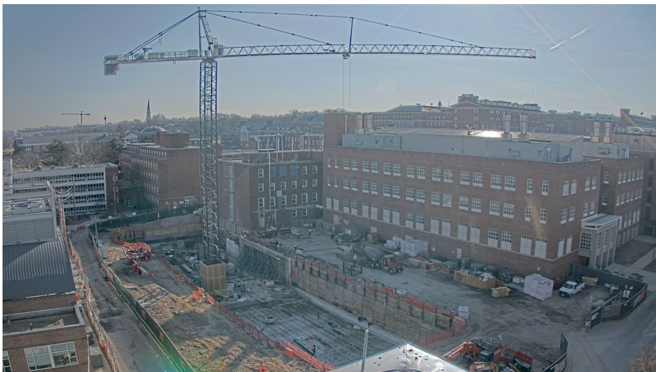
Photograph of construction activity (February 2022).
